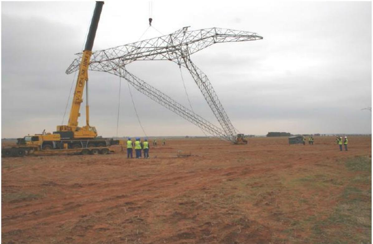
Figure 30. During construction of new infrastructure (Gyed V-pylons)<sup>9</sup>
